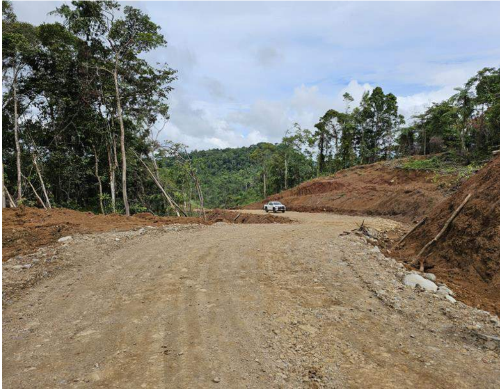
Section of the New Tolukuma Access Road
